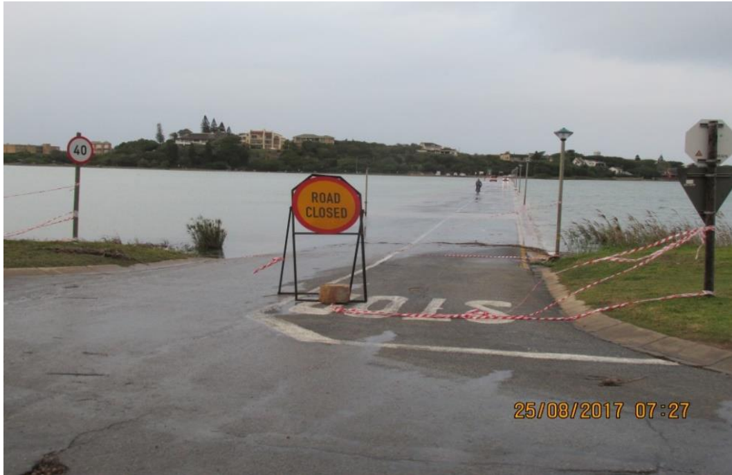
Plate 8 Berm overwash shown in Plate 6 resulted in the causeway overtopping with seawater. Zero freshwater inflow to the estuary occurred around this time, so that salinity levels in the estuary would remain at 35 or higher. High rates of evaporation would rapidly result in hypersaline conditions developing in the estuary as the estuary closed again within 48 hrs. Photo by Hennie Swanevelder – Department of Economic Development and Environmental Affairs.
