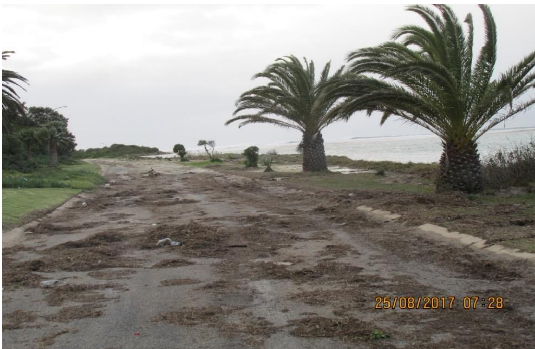
Plate 7 Berm overwash shown in Plate 6 deposited large quantities of flotsam on the Aston Bay road running parallel to the lagoon. Photo by Hennie Swanevelder – Department of Economic Development and Environmental Affairs.
