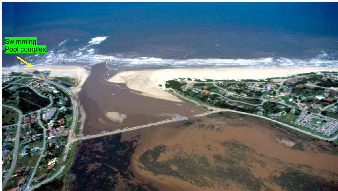
Plate 2 Construction of the carpark and then the swimming pool started in 1969. A stone embankment was also constructed on the western side of the carpark to stabilize the position of the estuary mouth. Consequently, the mouth channel was forced westwards and away from the shallower bedrock to the east. Breaking waves and the underlying slate beds can be clearly seen opposite the swimming pool. Forcing the mouth channel to the west enabled flood currents to erode deeper, draining the estuary at low tide (refer to photograph above). At the time of this photograph (probably mid 1980's), the original rubble causeway had been breached and floodwaters eroded a relatively deep and wide channel. The photograph also shows a plume of discoloured estuarine water radiating from the mouth – refer to Figure 5 (Photograph; T Wooldridge).
